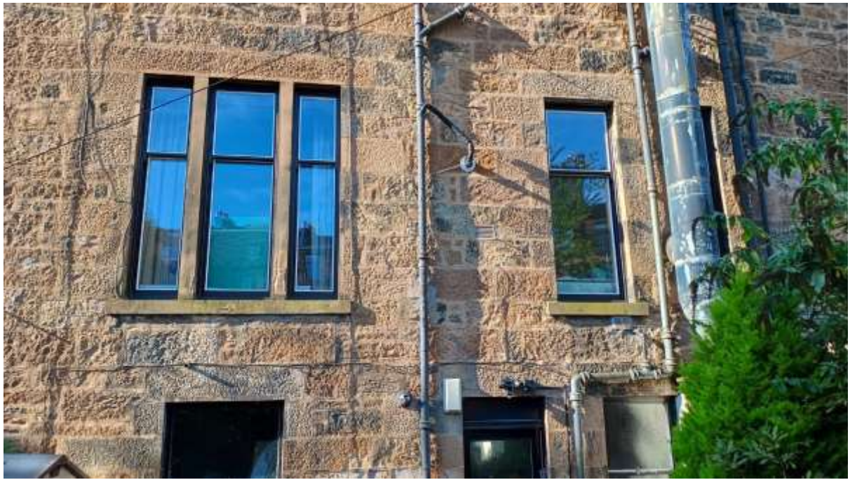
Replacement windows at rear
