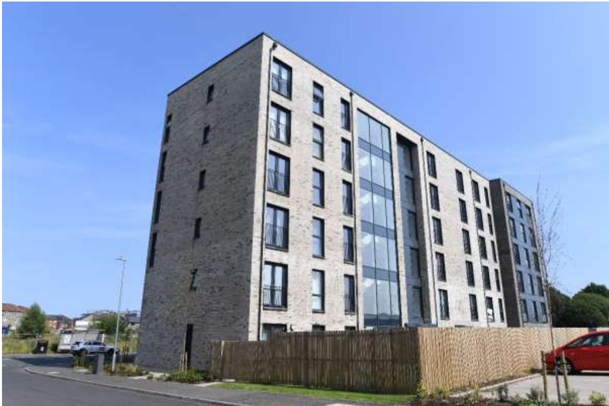
West of Scotland Housing Association – Dalmarnock Station
