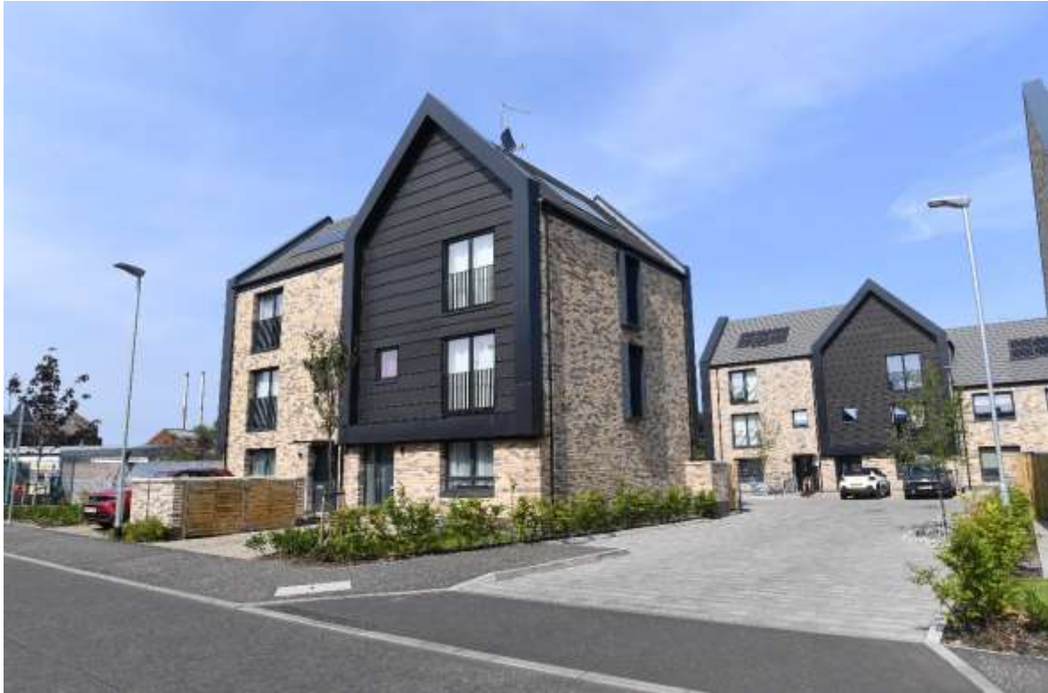
Link Housing – Dalmarnock Riverside Phase 3
