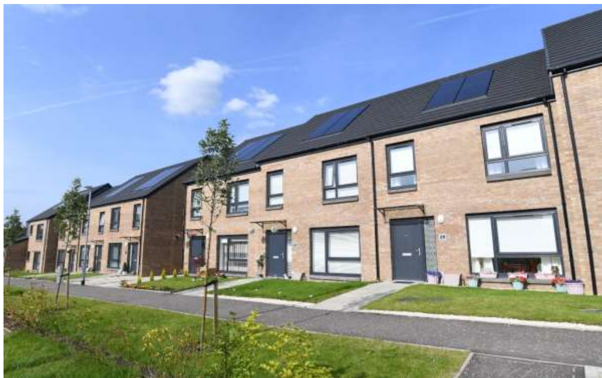
Calvay Housing Association – Garvel Crescent
