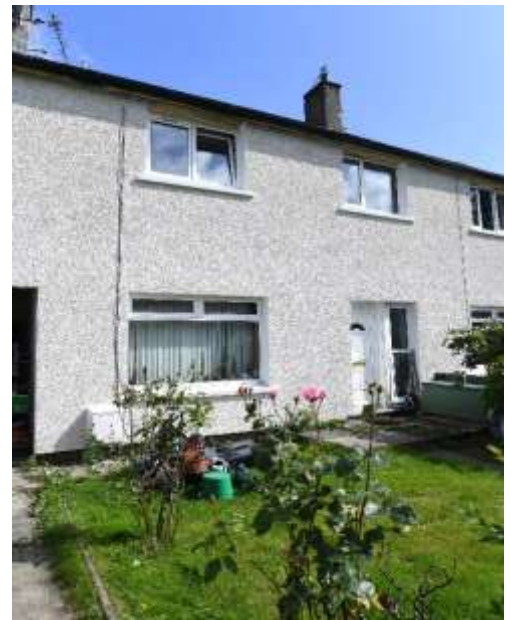
Figure 2. Angela's property in Kempsthorne after the EWI had been installed.
