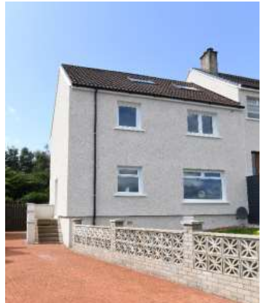
Figure 1. EWI works completed on Mrs Bell's property in Kempsthorne
