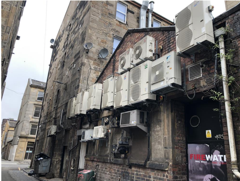
Photo 1: Numerous existing condenser units and kitchen extract flue from adjoining premises
