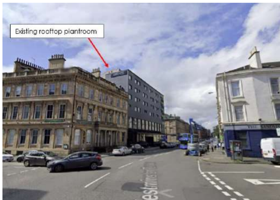
Figure 4: Existing rooftop plantroom as viewed from East near Westminster Terrace showing existing rooftop plantroom (Google Streetview May 2024)
