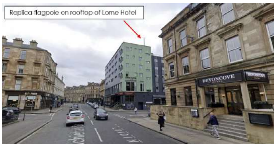
Figure 3: Existing Site from NW on Sauchiehall Street showing replica flagpole (Google Streetview May 2024)
