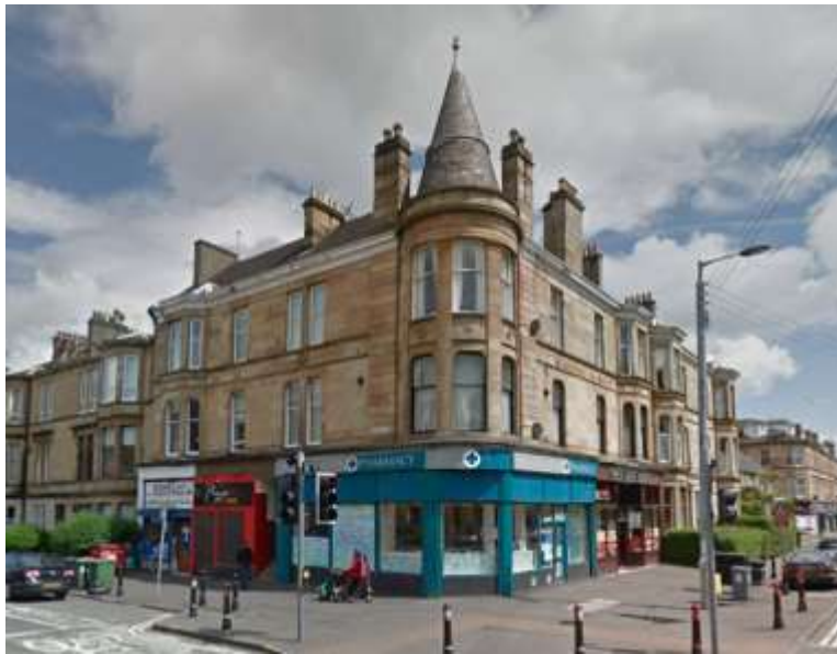
Figure 6: In 2017, prior to the fire, the building hosted four thriving businesses on the ground floor, including a pharmacy, with residences above.
