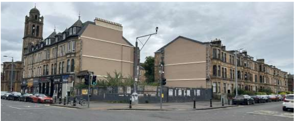
Figure 5: In 2025, six years since demolition in 2019 the site remains undeveloped and overgrown.
