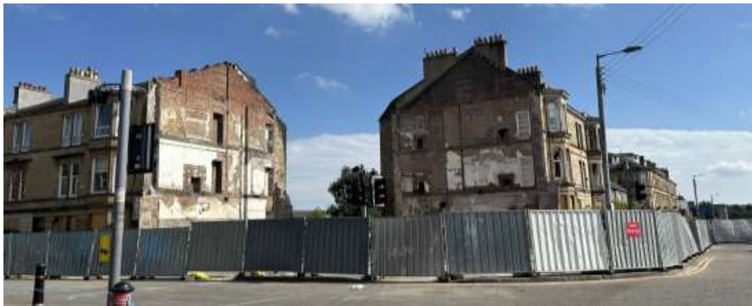
Figure 7: In 2025, post demolition, another big gap within the town centre
