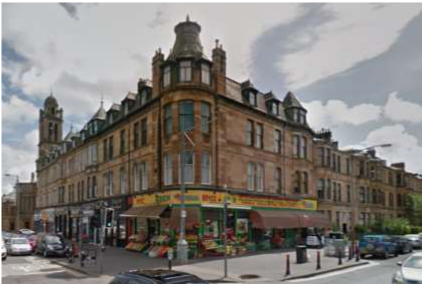
Figure 4: In 2017, prior to the fire, the building (property A) hosted three thriving businesses on the ground floor, including a corner grocery shop, with residences above.
