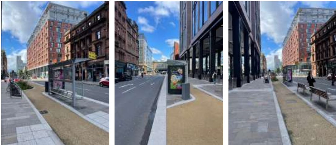
Completed exemplar section of Argyle St West
