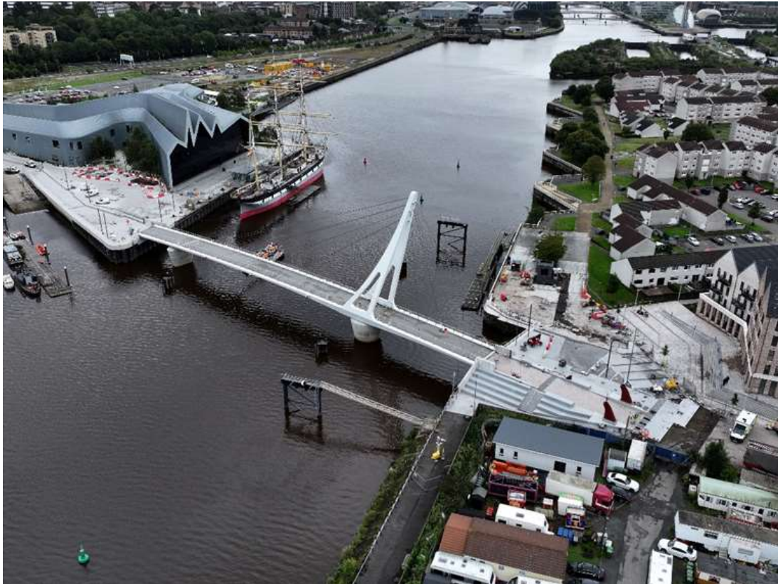
Aerial View of Govan / Partick Bridge during construction.
