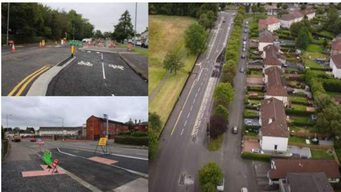
Varying images from the construction of NEATR Phase 1
