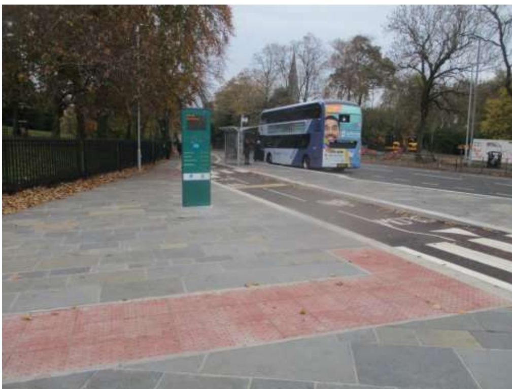
Completed floating bus stop on Grange Road within Phase 1 of Connecting Battlefield
