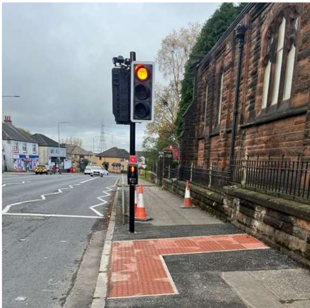
Improvements at Balmore / Knapdale Pedestrian Crossing
