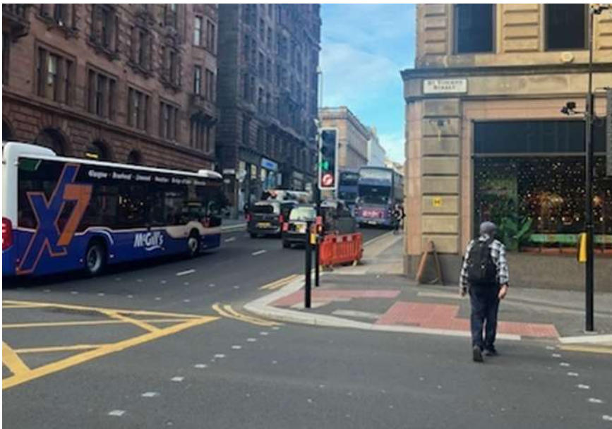
Improvements at St. Vincent Street Junction
