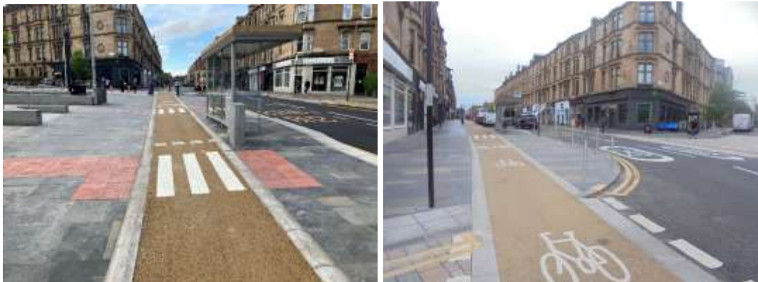
Images showing completed works on Byres Road.
