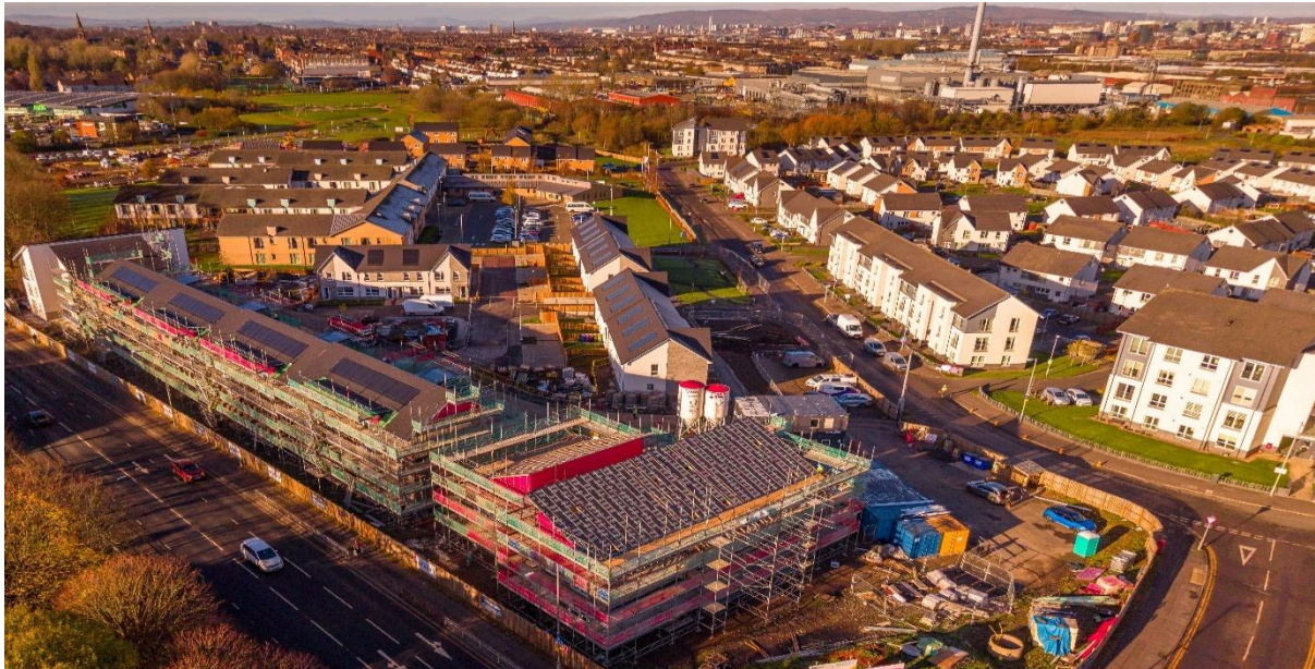
North Toryglen TRA- Kings View (Final Housing Phase)
