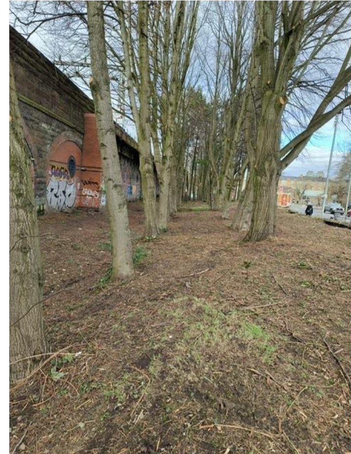
Bridge Street litter removal & vegetation cutback (March 2026)
