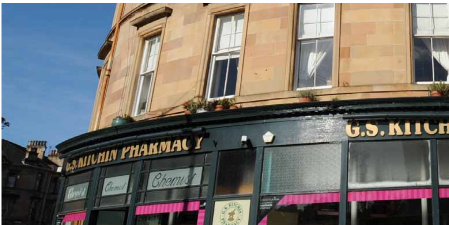
1 View of the south west building on Kenmure Road
